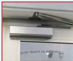
Reinforced for Arm Closer
